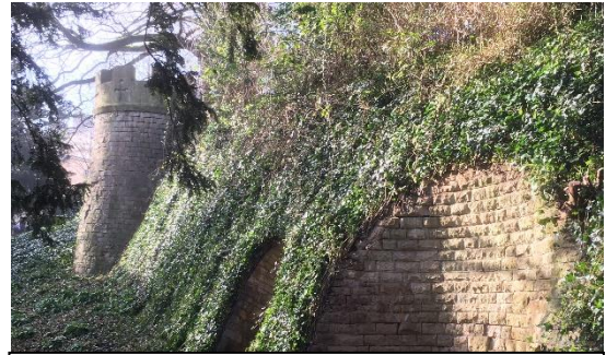
Great Retaining Wall & Battlement Tower ( HE Listed )
